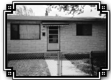
245 N. 3 rd , built 1907. Roy Yokota's home.
