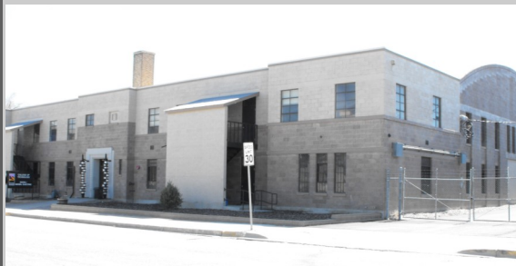
1. Idaho State University College of Technology Diesel/Electric 1235 S. Second
