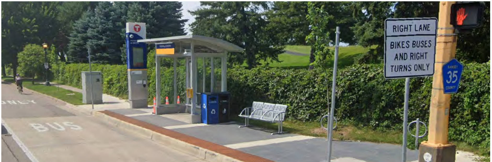
Existing bus stop at 4th Avenue and Lovejoy Street (top); example of a highly amenitized bus stop, including shelter, seating, trash and recycling receptacles, transit stop marker/sign with schedule, bike racks, raised curb, and specialized paving. Enhanced stops could include any combination of these elements, depending on location, available space and ridership (bottom). Source: Google Earth
