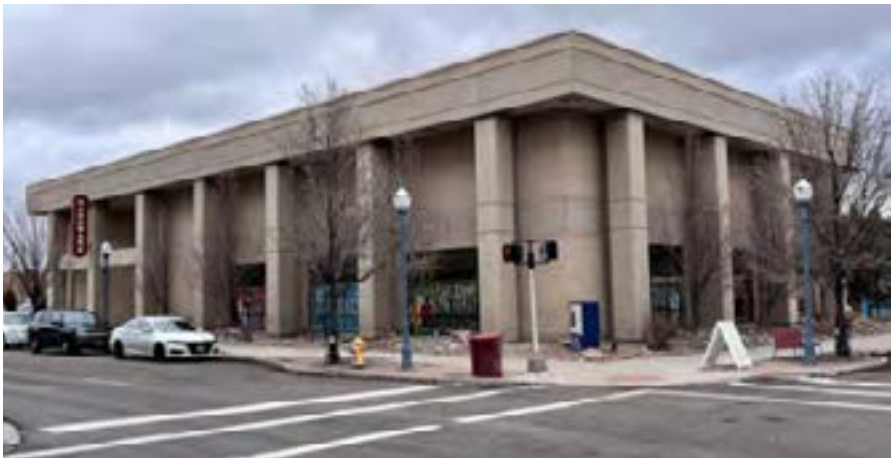
Commercial Building, 120 N. Arthur Ave., Brutalist, 1981.
