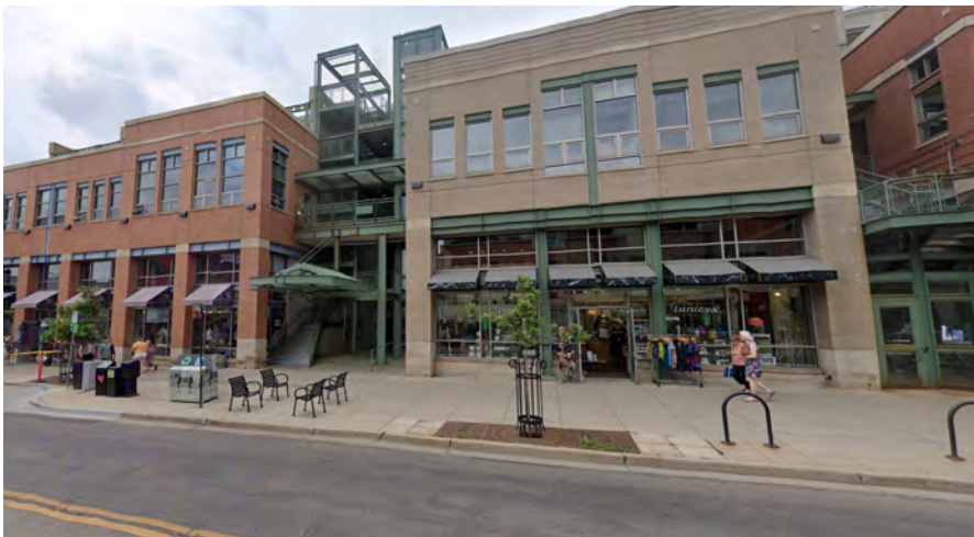
Parking structure lined with retail buildings. Source: Google Earth
