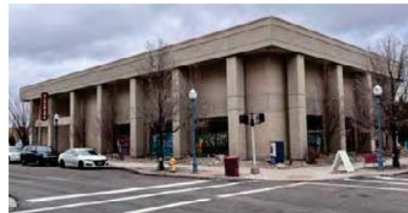
Commercial Building, 120 N. Arthur Ave., Brutalist, 1981.
