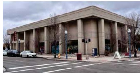
Commercial Building, 120 N. Arthur Ave., Brutalist, 1981.
