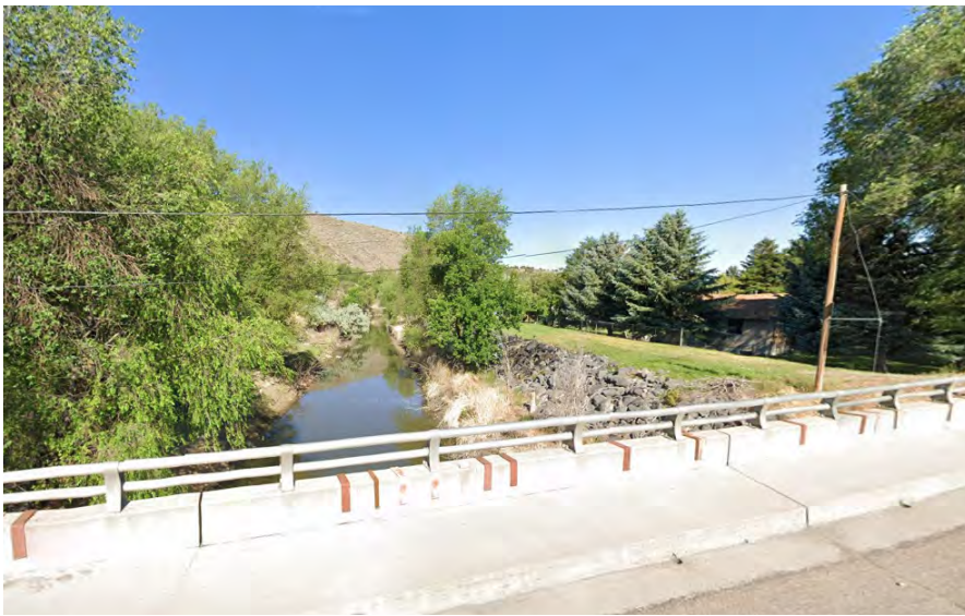
View of Portneuf River and levee structure at Bannock Hwy bridge crossing. Source: Google Street View
