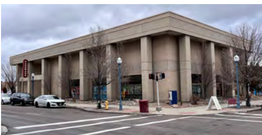
Commercial Building, 120 N. Arthur Ave., Brutalist, 1981.
